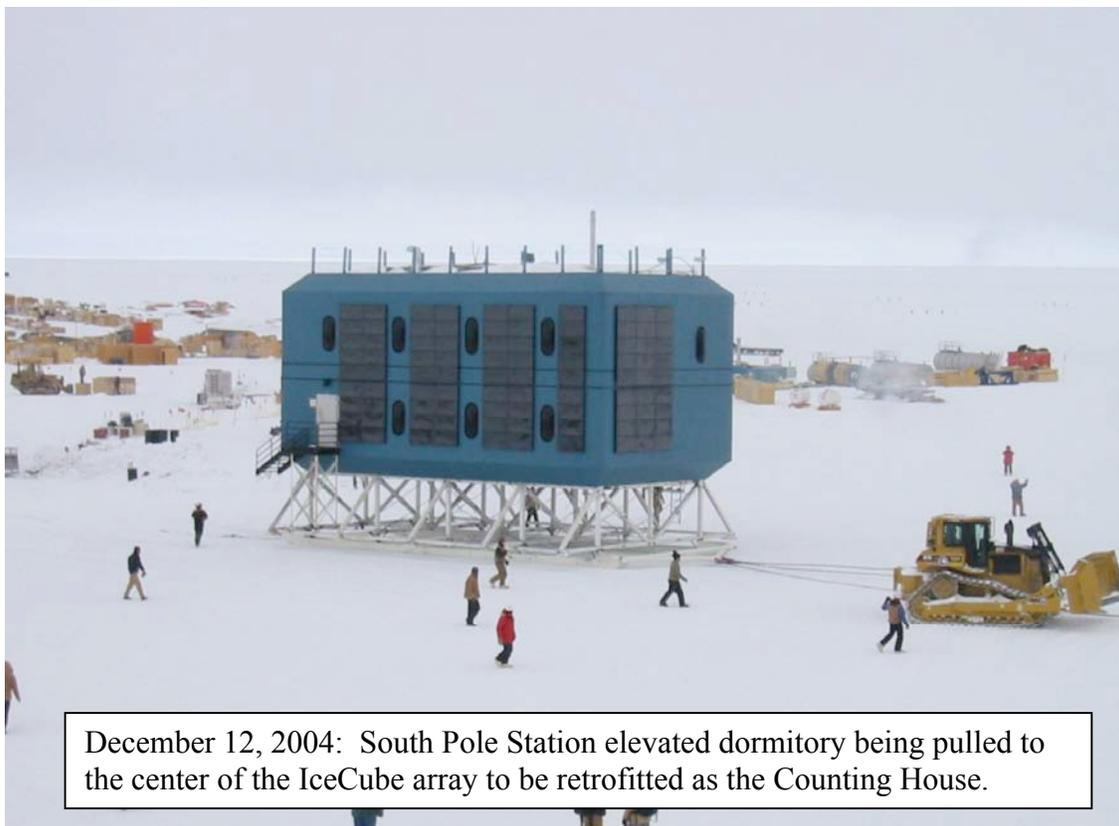
December 12, 2004: South Pole Station elevated dormitory being pulled to the center of the IceCube array to be retrofitted as the Counting House.
